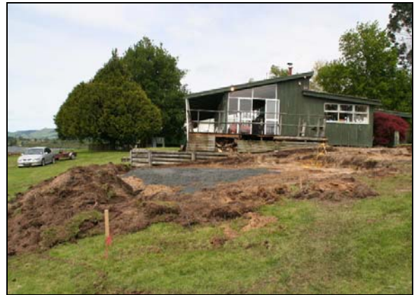
Excavations for new BBQ complete
