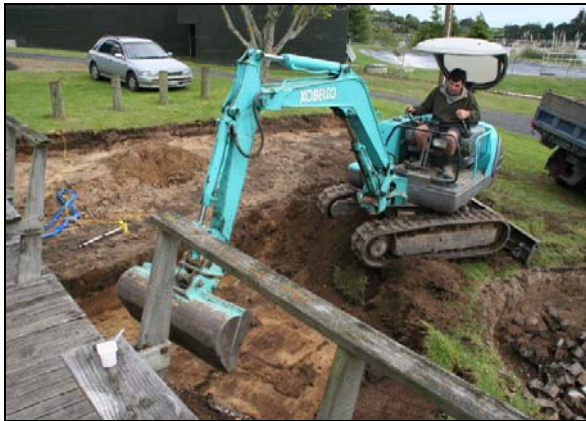
Excavations for new BBQ started
